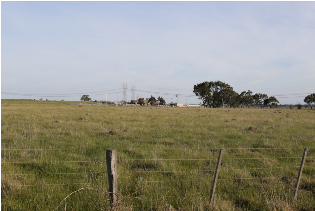
Figure 14-15 Wollert Compressor Station from Summerhill Road (located at VP16)
