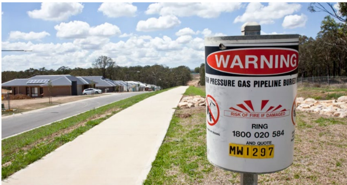
Figure 14-10 Example of a pipeline marker
