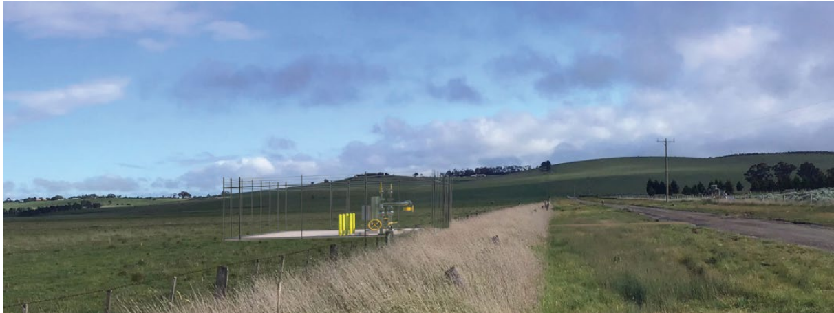
Figure 14-14 Photomontage: predicted view of MLV3 at Gunns Gully Road (located at VP12)
