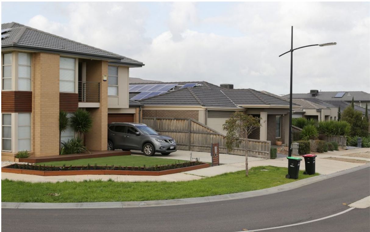
Figure 14-7 View south-west of dwellings along Inkerman Crescent, Mickleham
