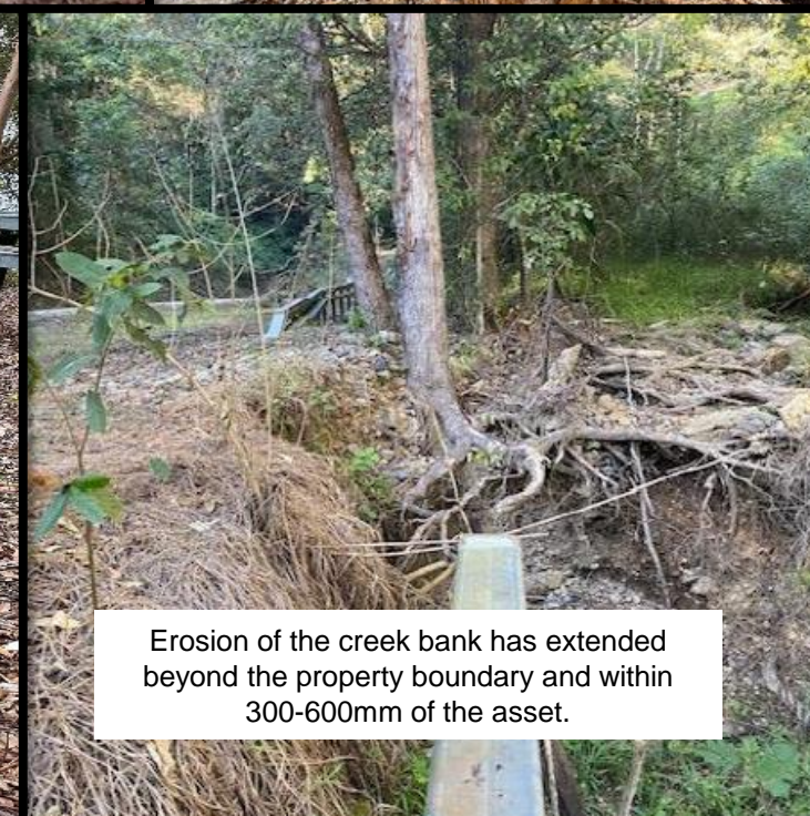
Erosion has continued impact the creek bank and has now undermined the asset
