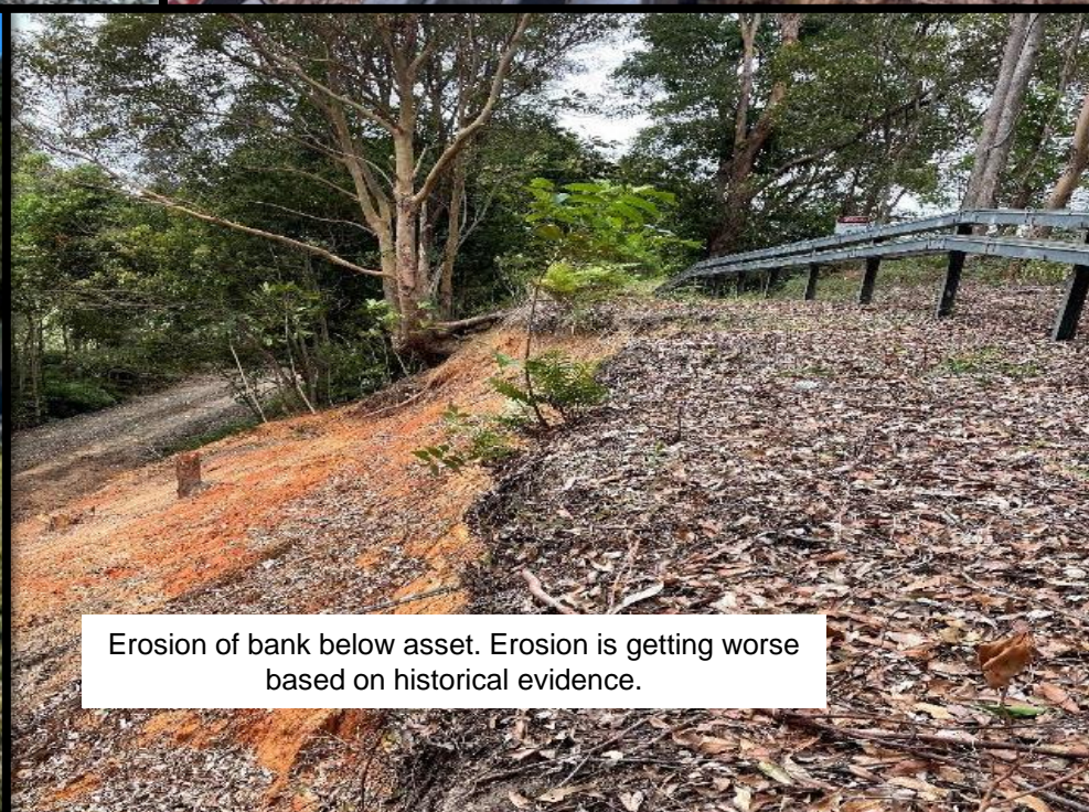
Erosion of the existing overland flow path has extended towards the electrical poles & the stays, potentially compromising the asset. The distance between the edge of the erosion and electrical pole is 6.14m. The shallow water table is further impacting the erosion of the surrounding ground.
