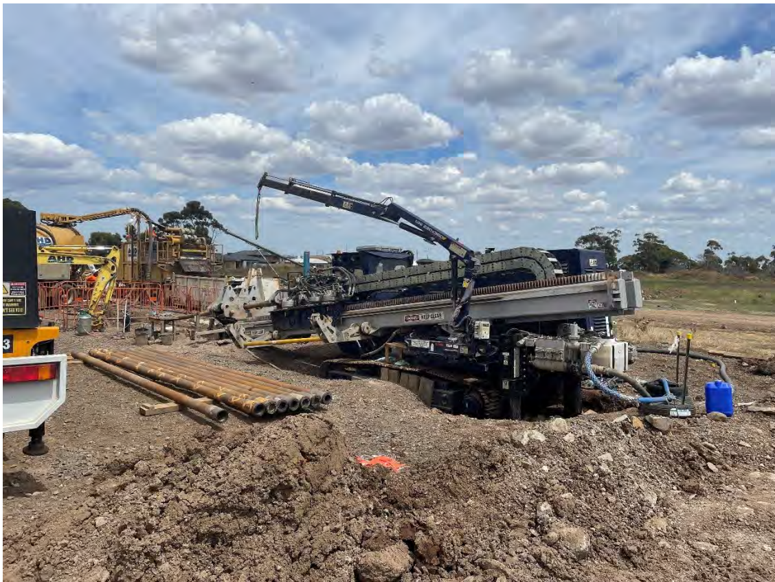
KP3.3 HDD at Melton Highway – HDD rig
