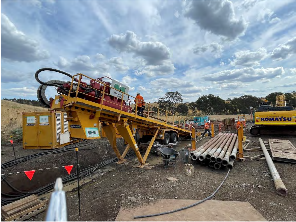
KP16.8 HDD at Deep Creek – HDD rig
