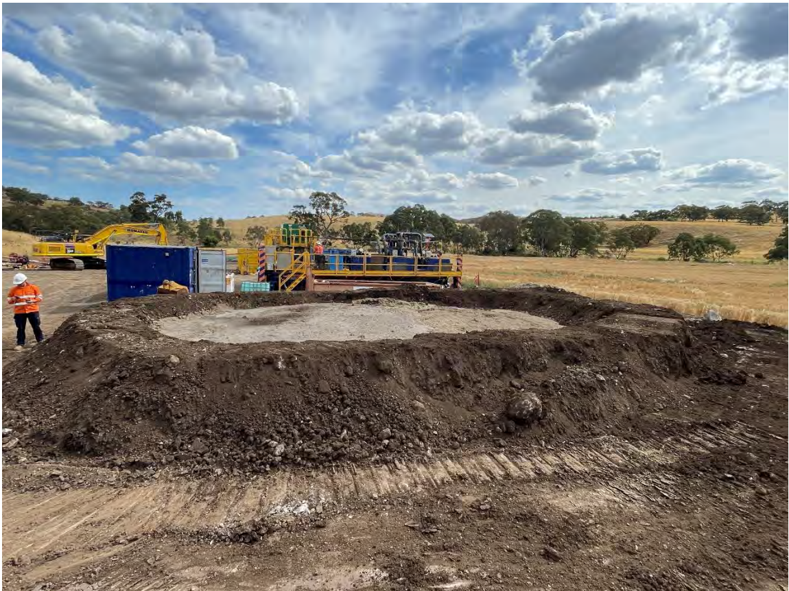
KP16.8 HDD at Deep Creek – mud sump using earthen bund
