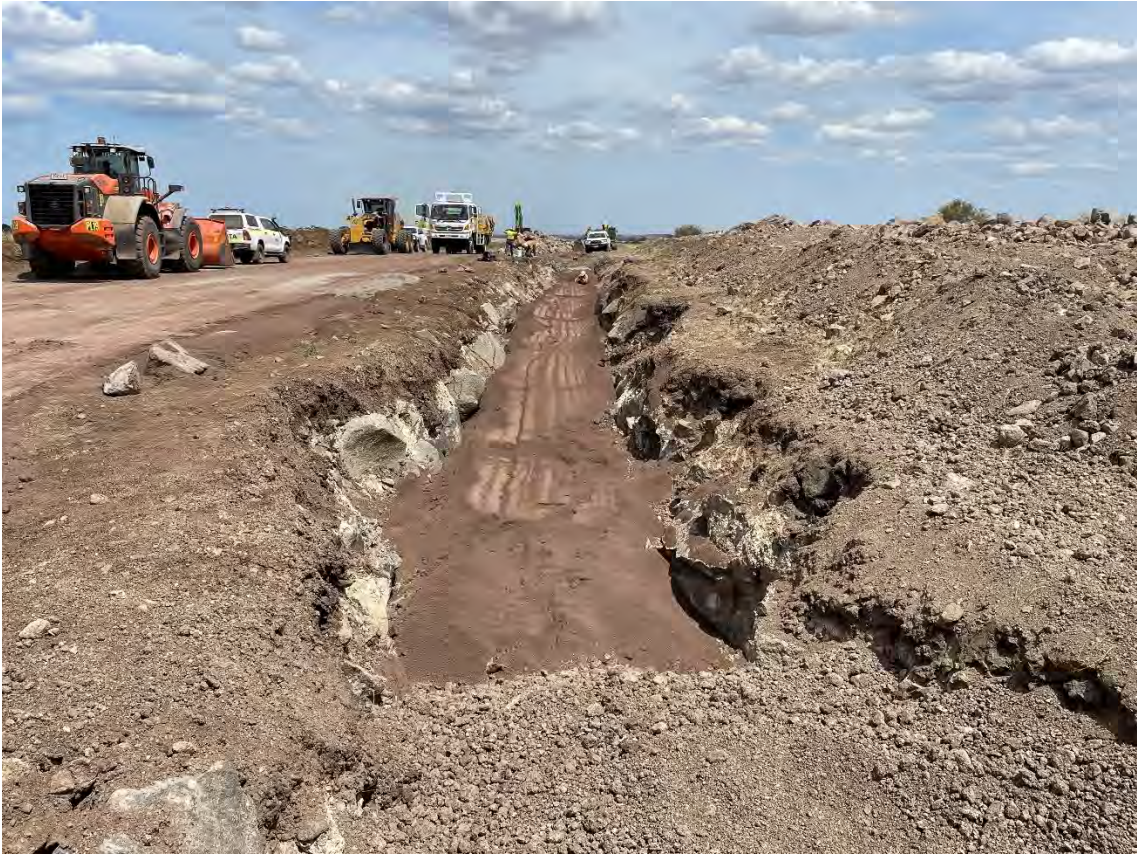
KP5 – soil fines reinstated in the trench prior to topsoil reinstatement
