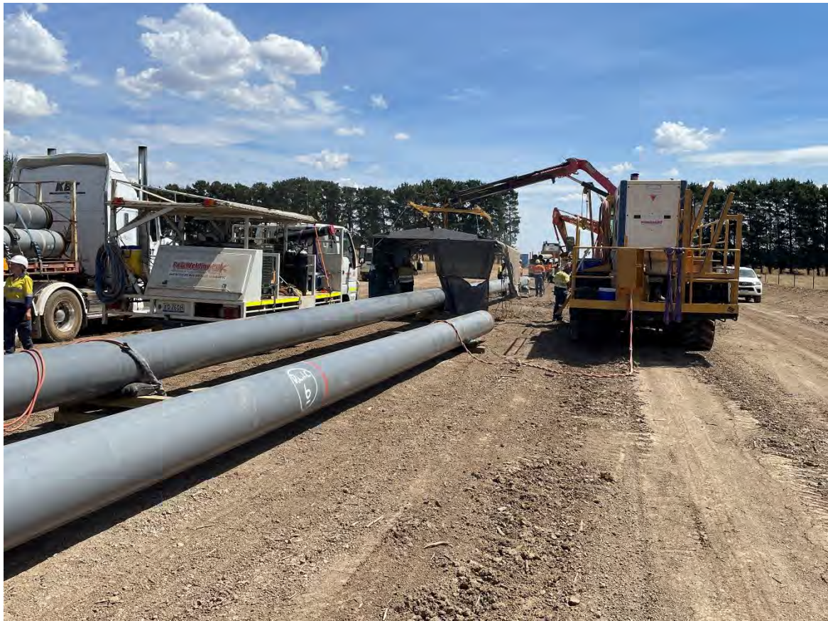
KP39.1 Donovan's Lane – pipe welding over the cleared RoW
