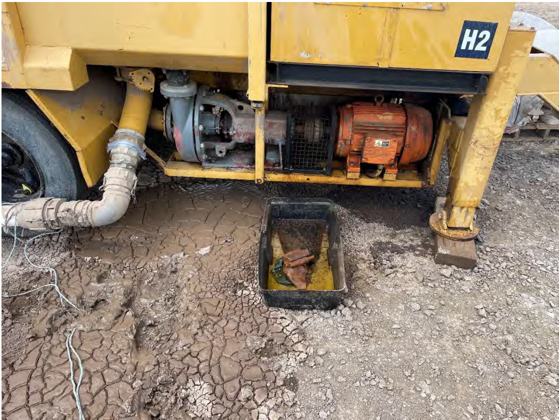
KP3.3 HDD at Melton Highway – drip tray used under generator
