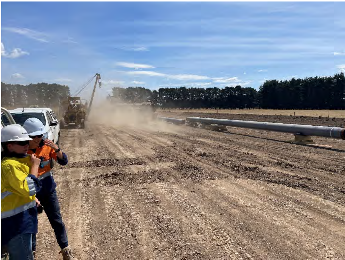
KP39.1 Donovan's Lane – dust generation from the pipe string truck
