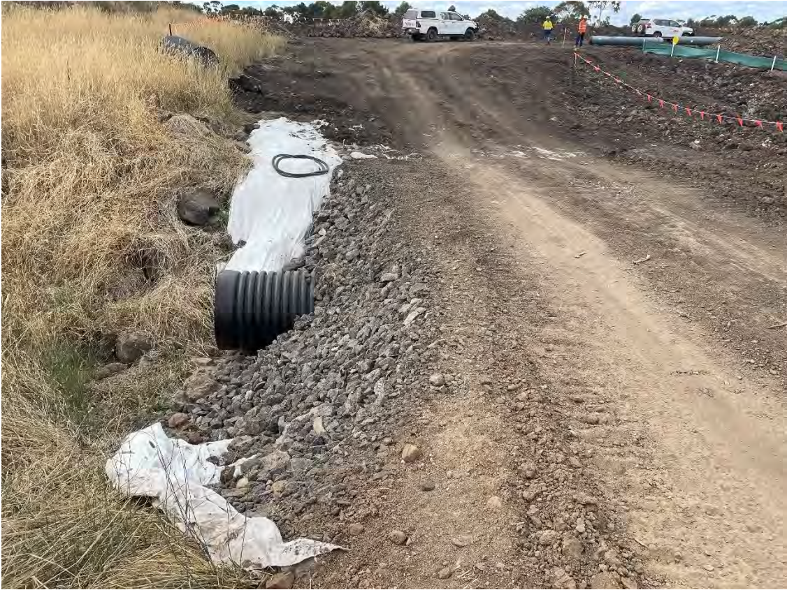
KP10.5 Unnamed tributary of Jackson's Creek – view across creek crossing
