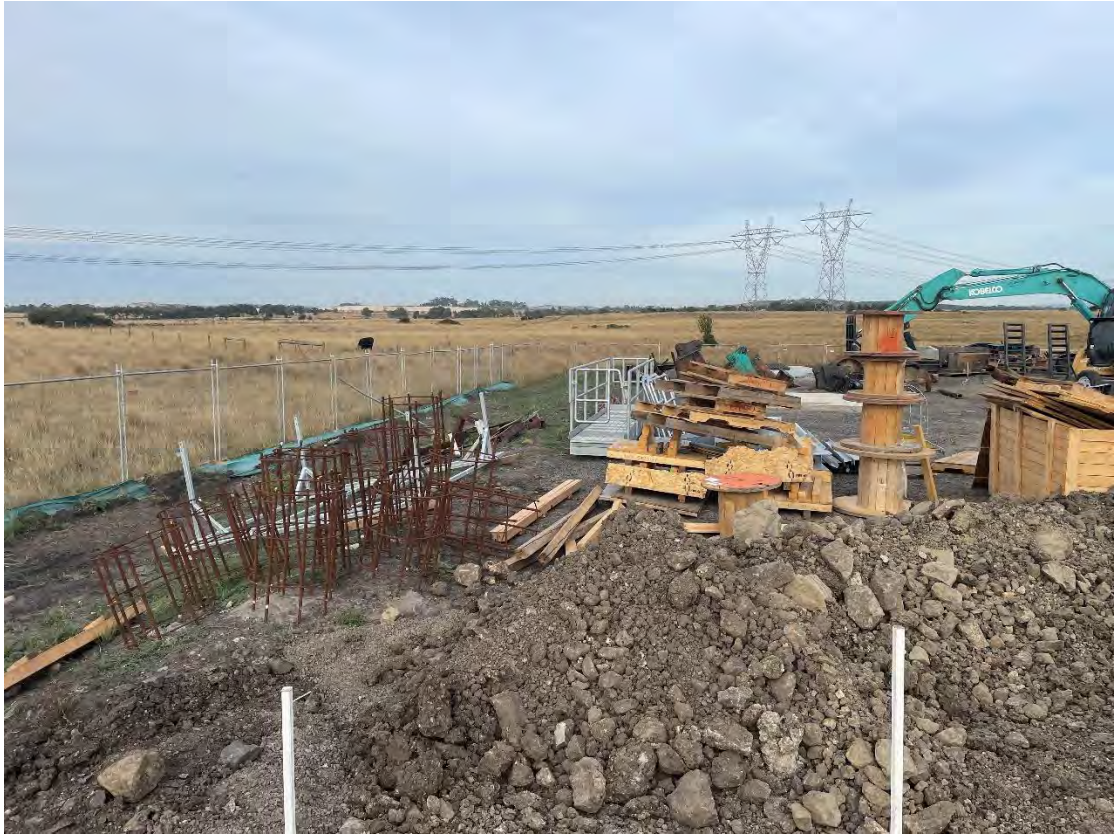
Compressor station – laydown area
