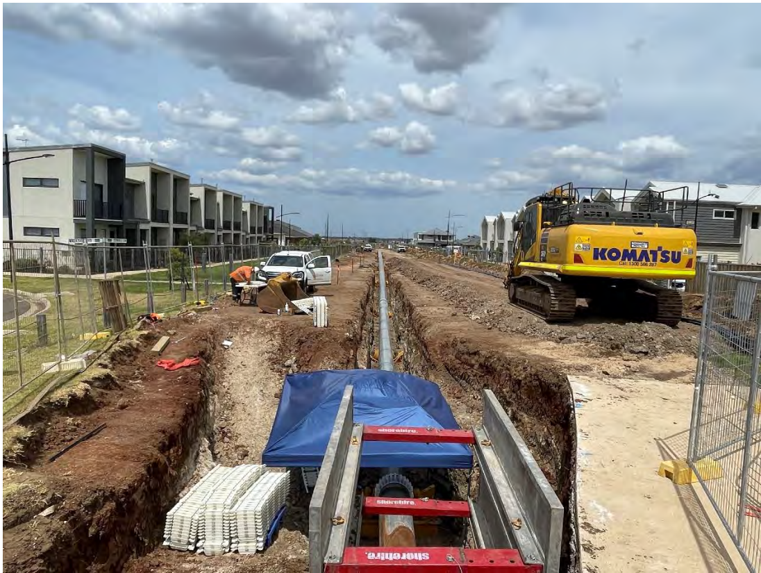
KP2 – boring under park in new residential area
