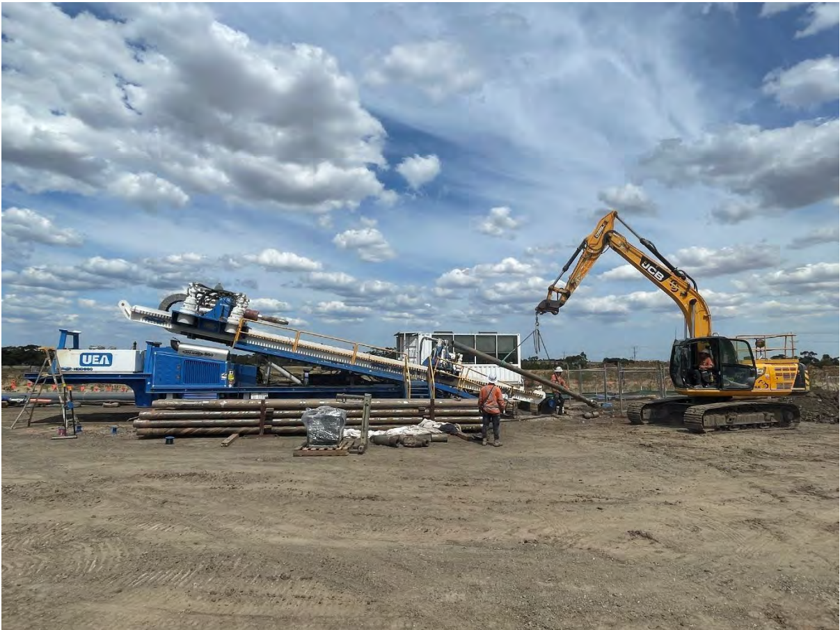
KP5 – pipe joint coating without the use of drip mats
