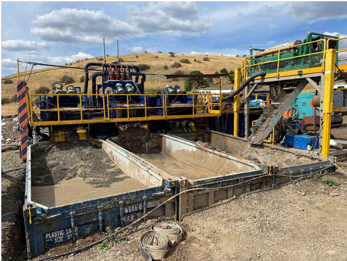
KP16.8 HDD at Deep Creek – cuttings treatment
