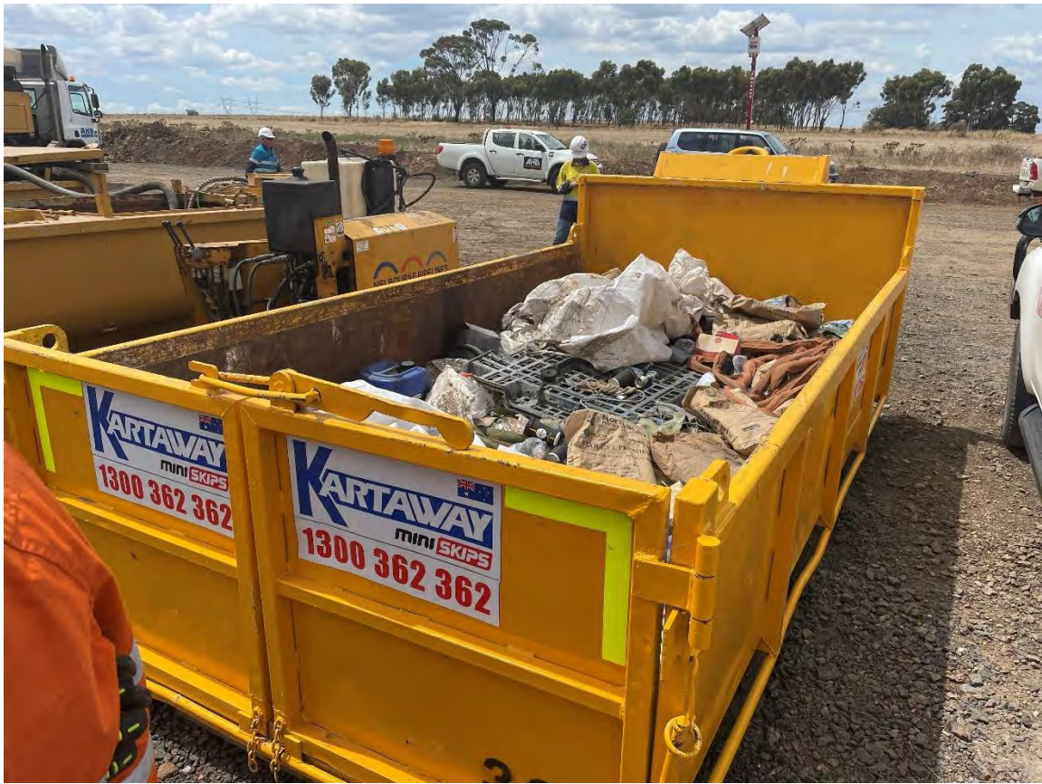
KP3.3 HDD at Melton Highway – general waste skip
