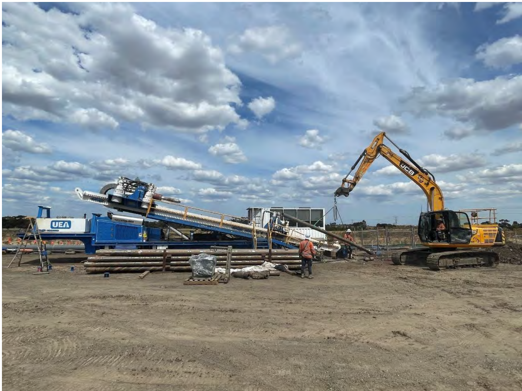
KP8.8 HDD at Calder Highway – HDD rig
