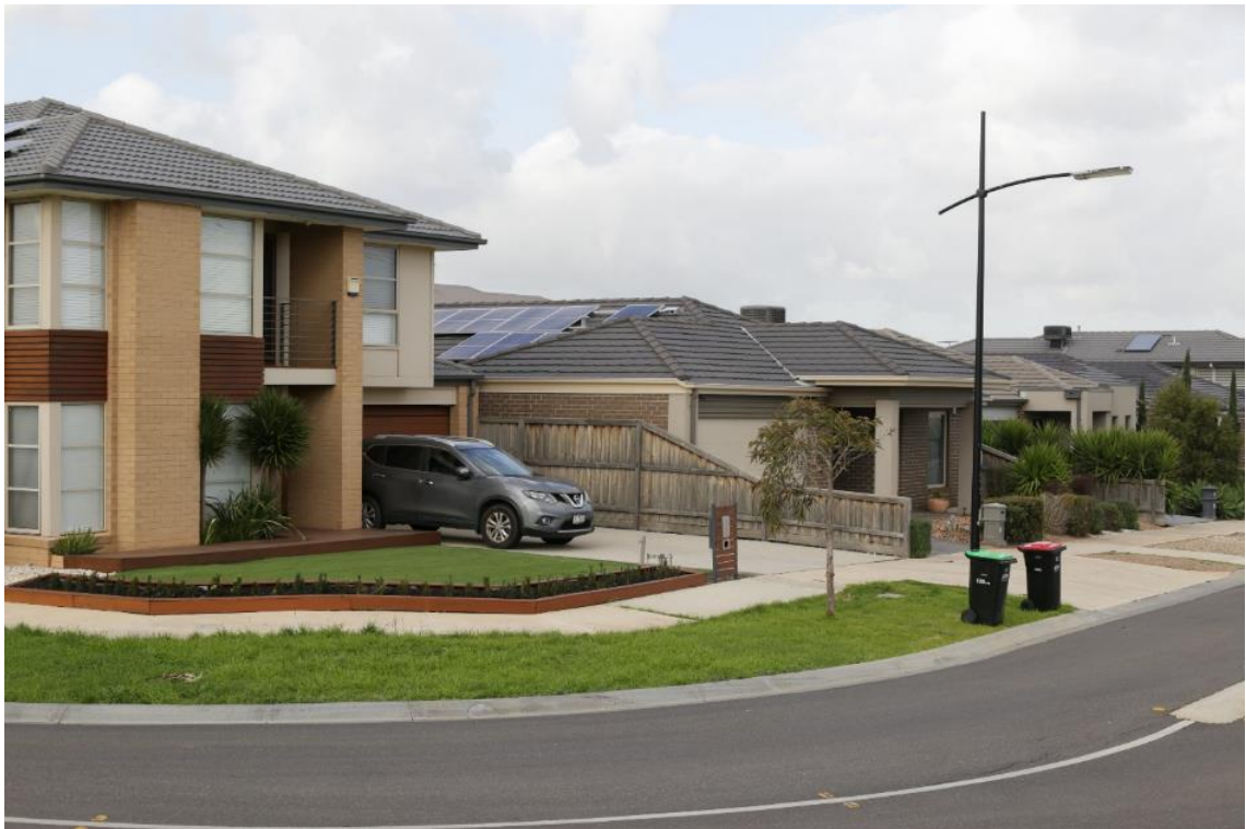
Figure 19 View south-west of dwellings along Inkerman Crescent, Mickleham
