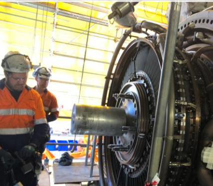
Gas turbine disassembled during the overhaul at DPS
