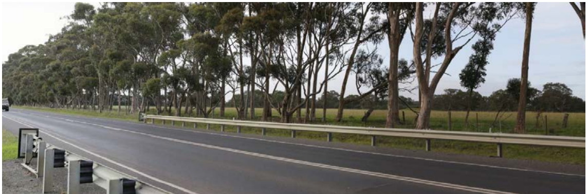
Figure 27 View north-west along Oaklands Road
