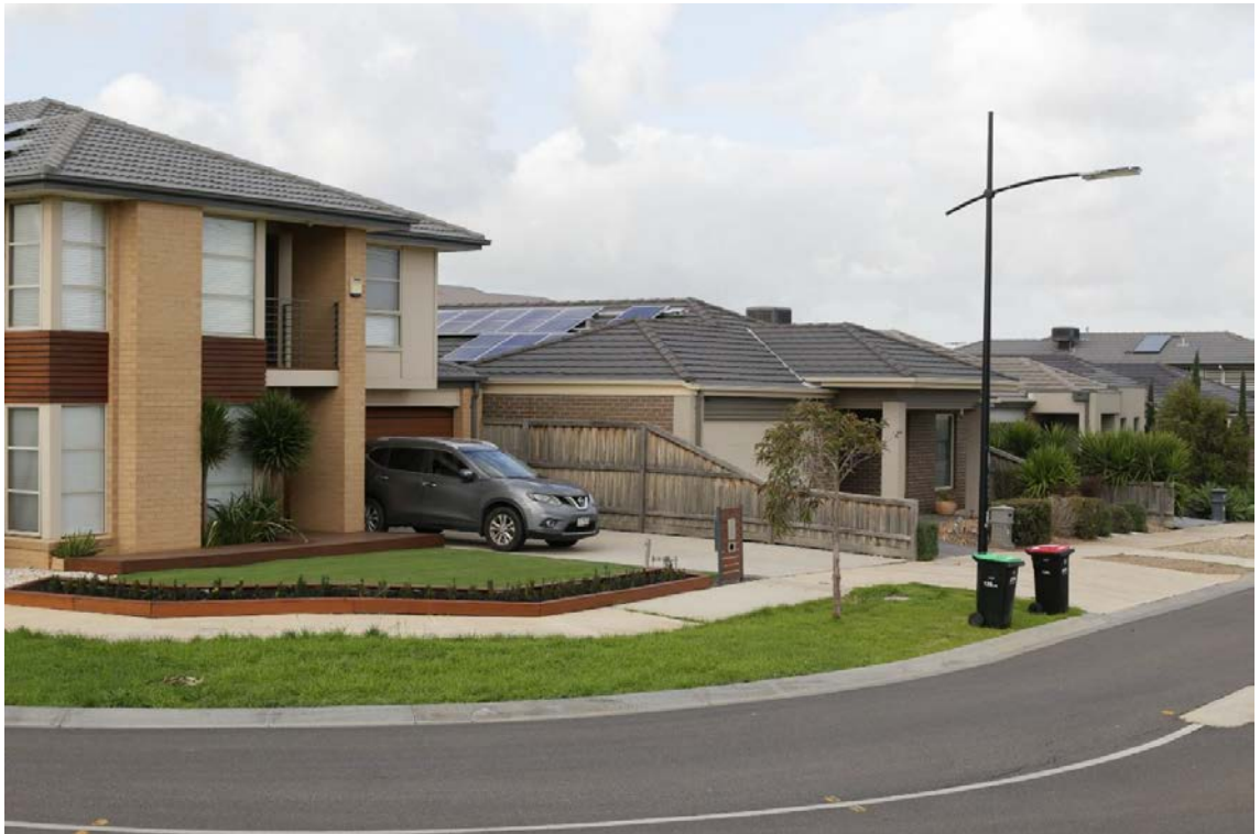
Figure 15 View south-west of dwellings along Inkerman Crescent, Mickleham
