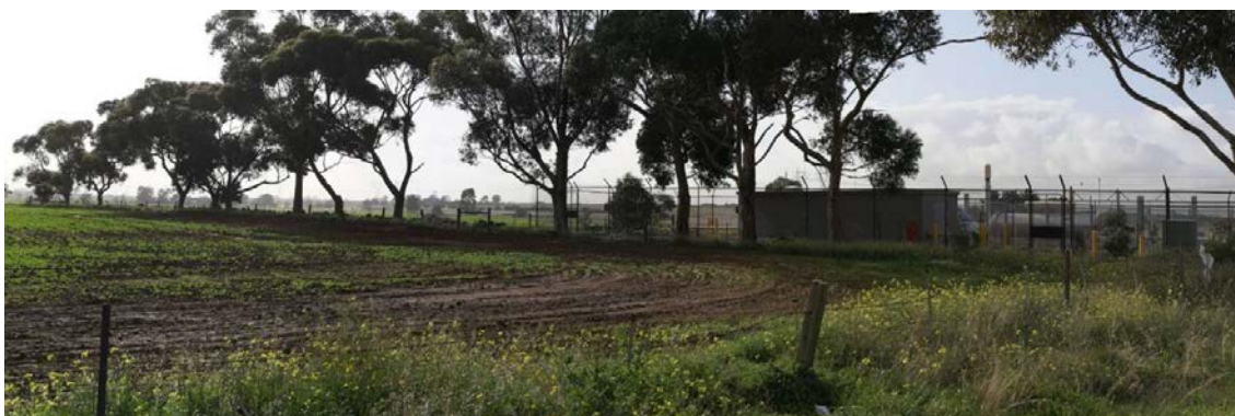
Figure 19 View north-west from Taylors Road towards the Plumpton Regulating Station
