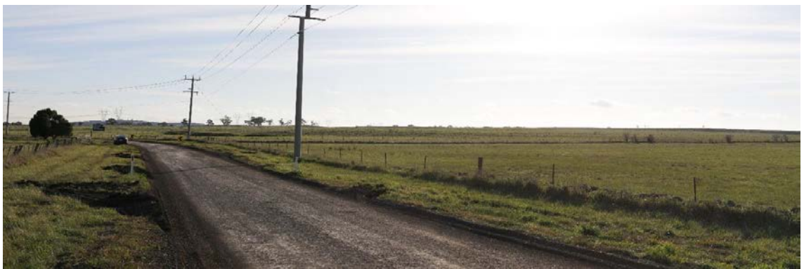
Figure 36 View south along Summerhill Road
