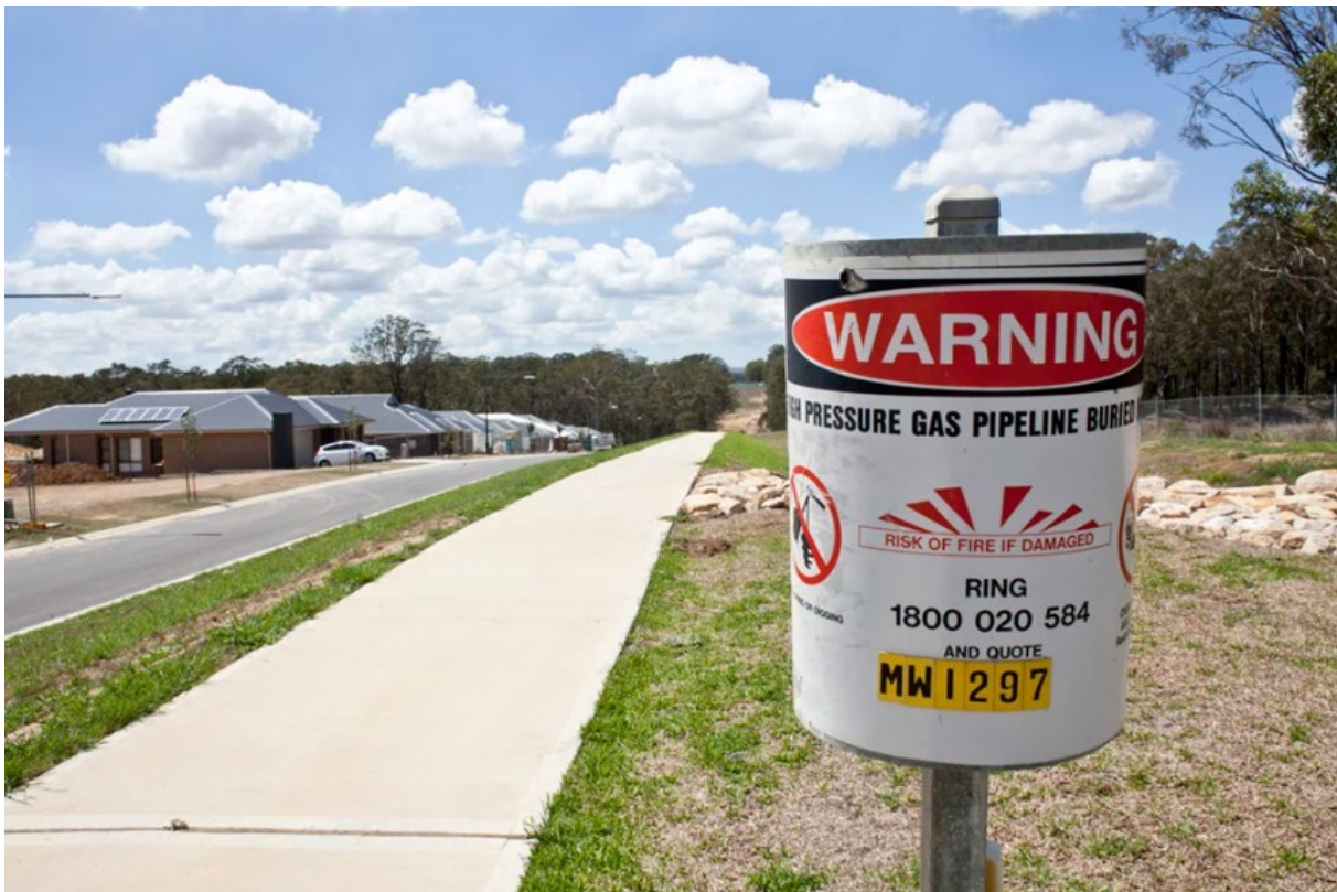
Figure 4-5 Example of a pipeline marker
