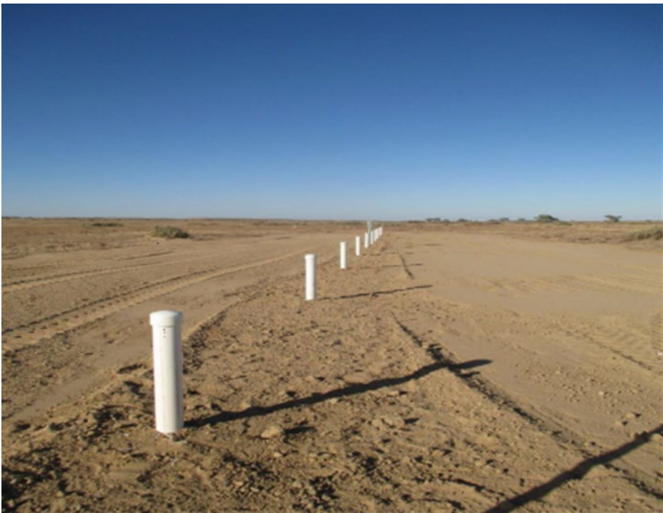
Figure 4-4 Cathodic protection anode bed PVC stand pipes, chimneys, or upstand test points
