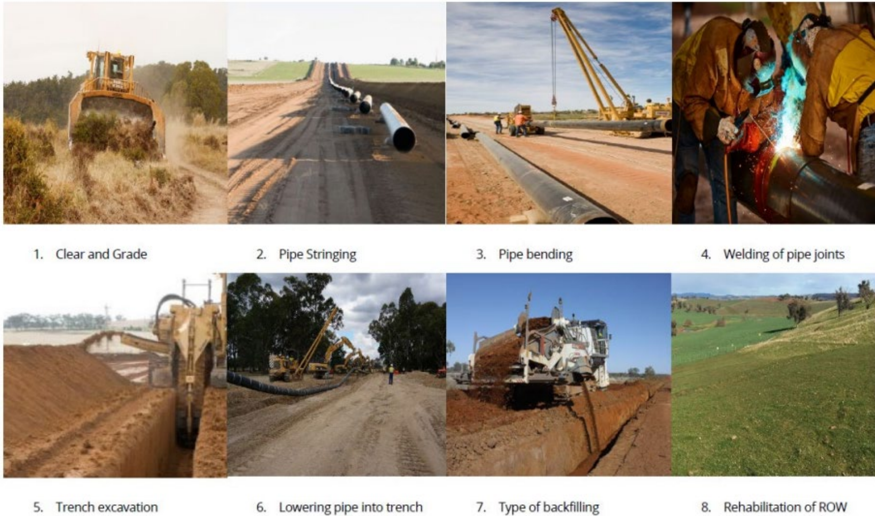
Figure 4-10 Pipeline construction sequence
