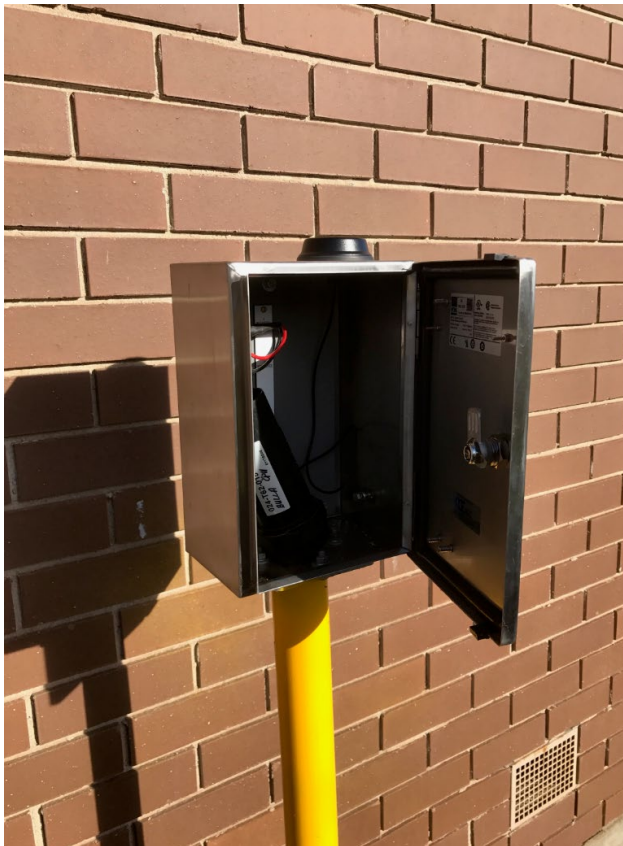
Figure 4-2 Typical Impressed Current Cathodic Protection (ICCP) system
