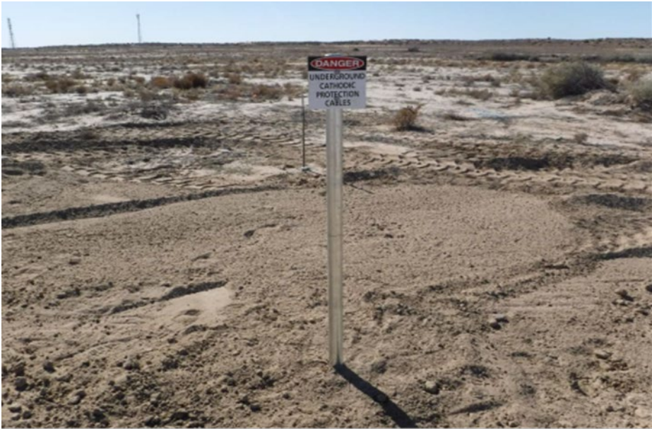
Figure 4-4 Cathodic protection anode bed PVC stand pipes, chimneys, or upstand test points
