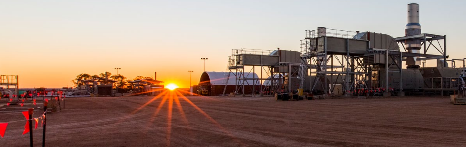
Sunset over Wallumbilla Gas Hub, Queensland.
