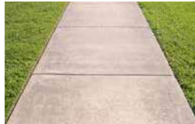
Broom finish concrete
