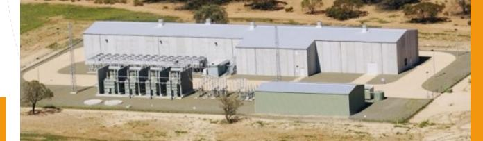
Murraylink uses Hitachi (ABB) generation 2 IGBT technology
