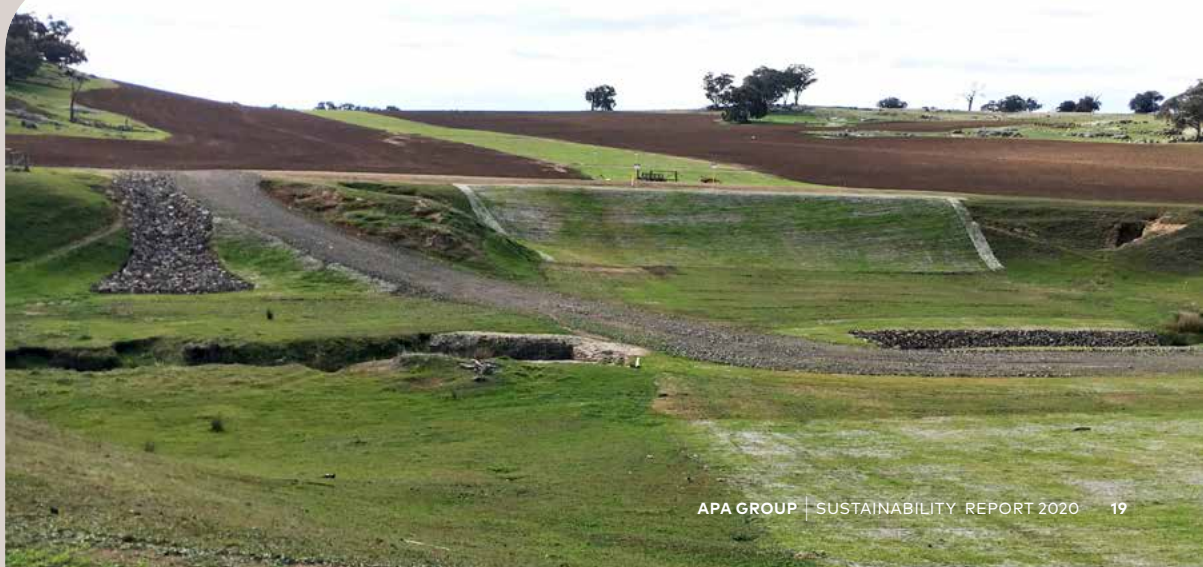
Restored easement after pipeline construction.
