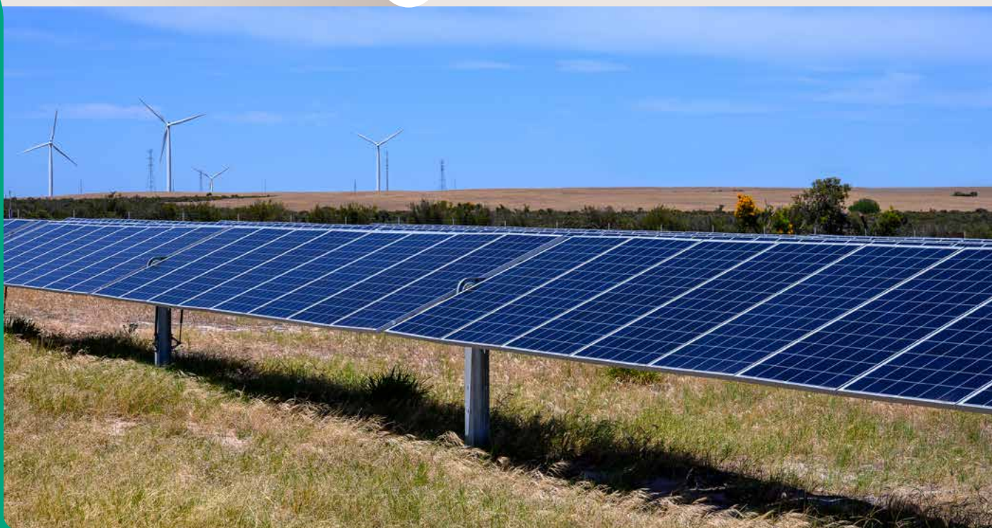
Badgingarra Solar Farm, with the Wind Farm in the background.
