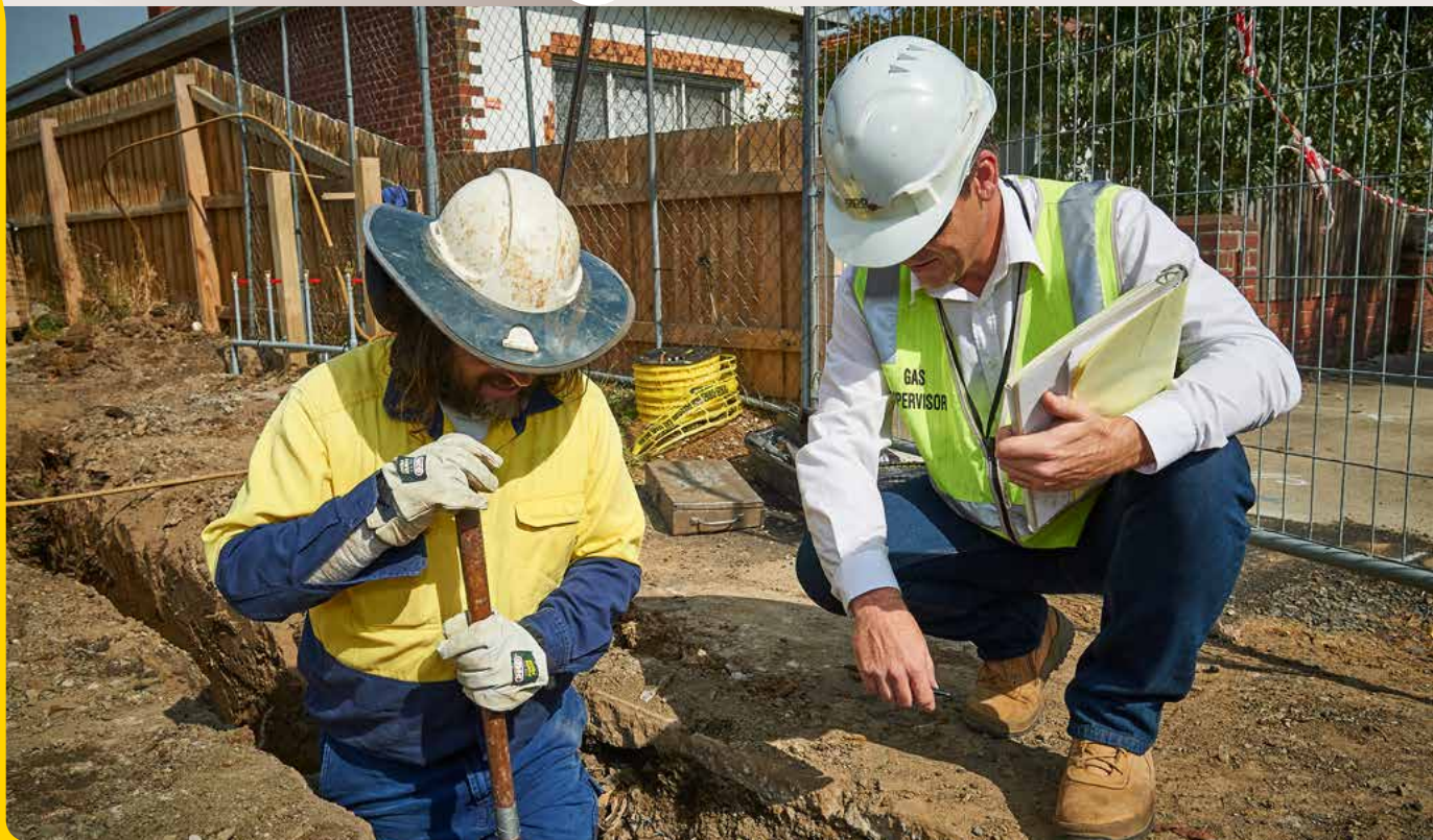
APA Field Supervisor onsite to ensure safe construction around pipelines.
